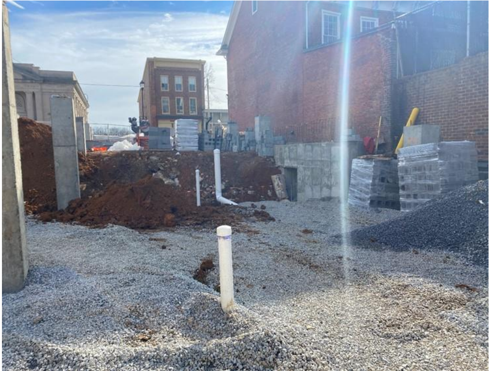
Backfilling and stone placement
