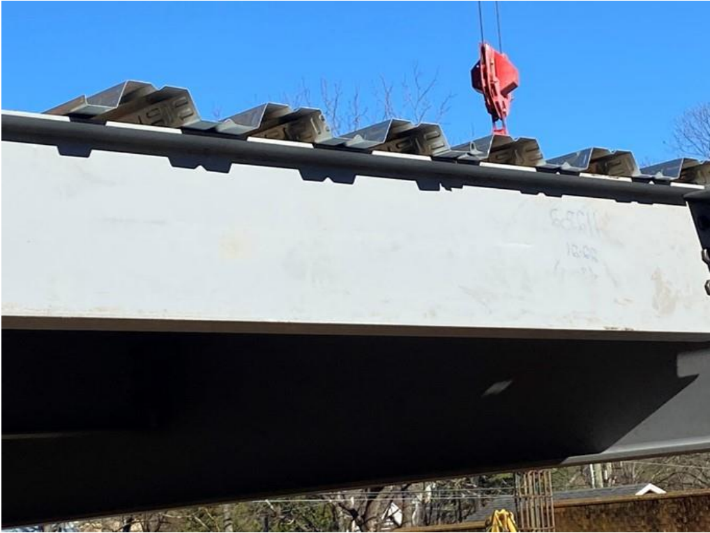
Decking install for sequence 1
