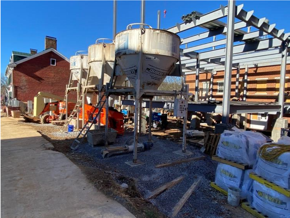
Mason setting up silo for mixing mortar and grout
