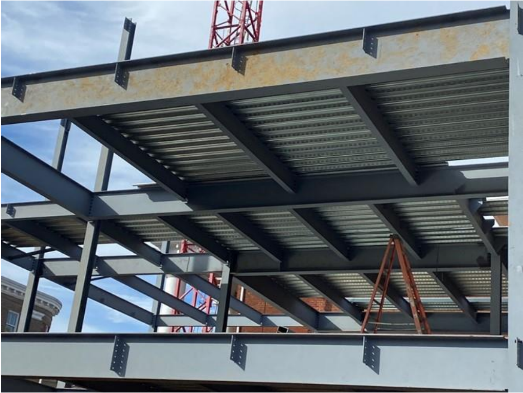
Welding and decking install for sequences 1&2
