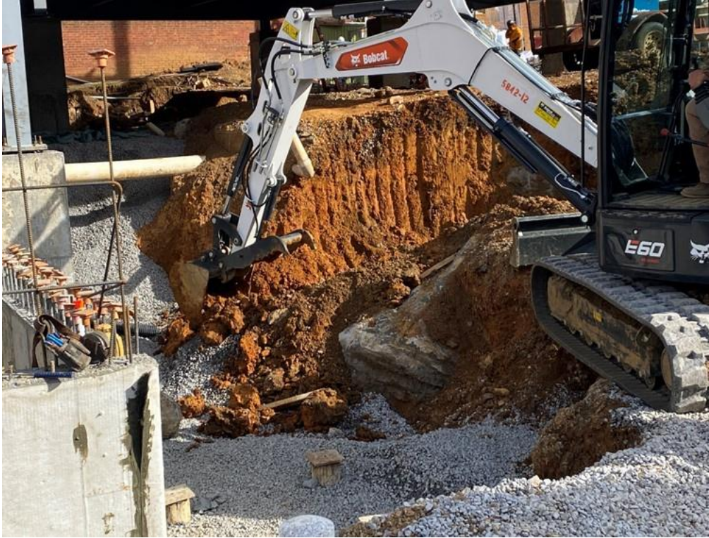
Excavation for equipment and electrical rooms foundations
