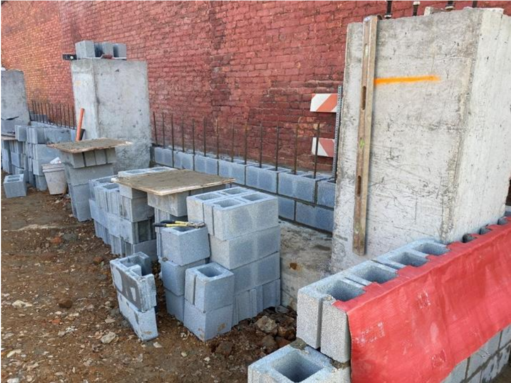
CMU wall installation on XA line
