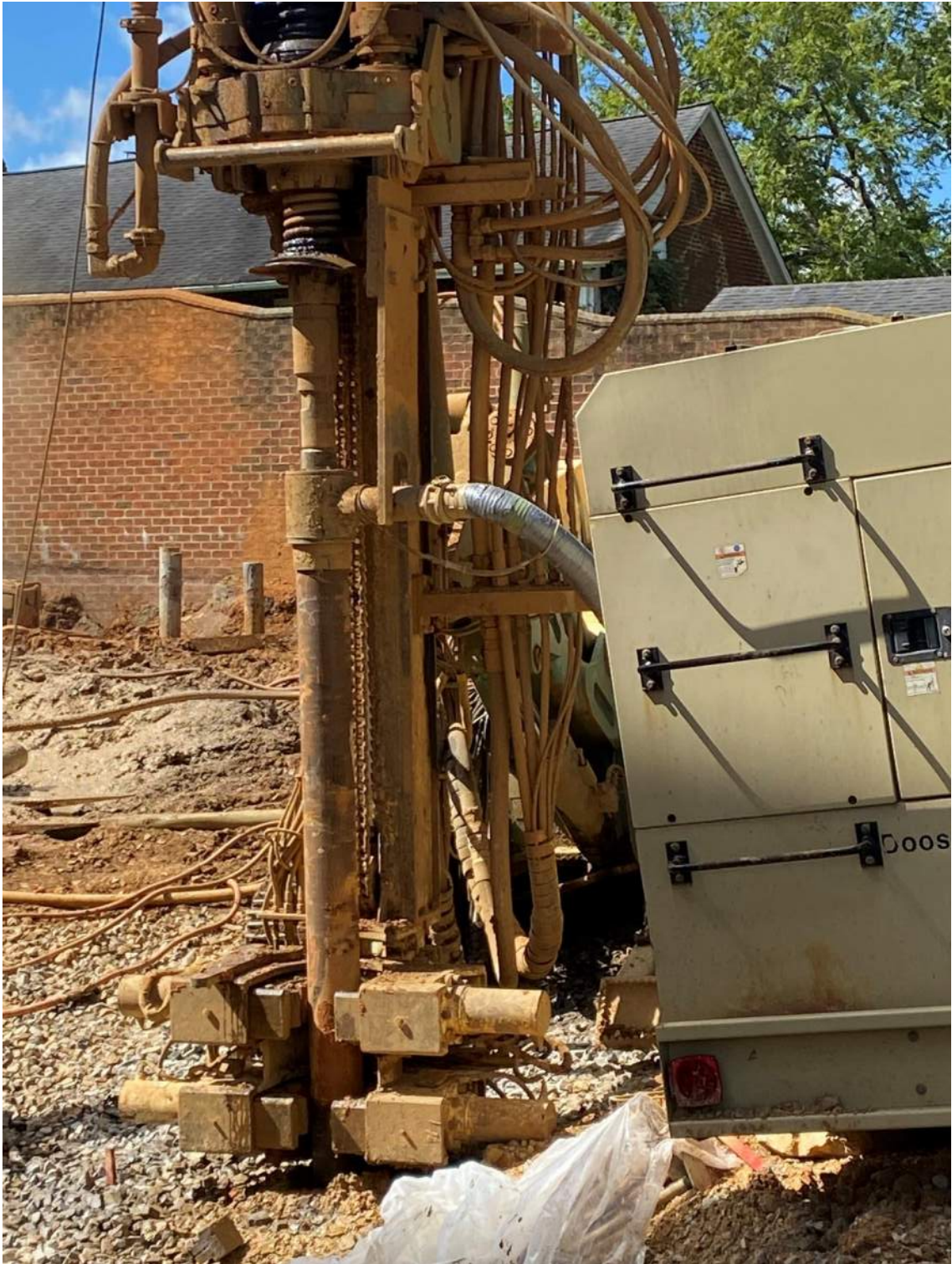
Micro pile installation, continued
