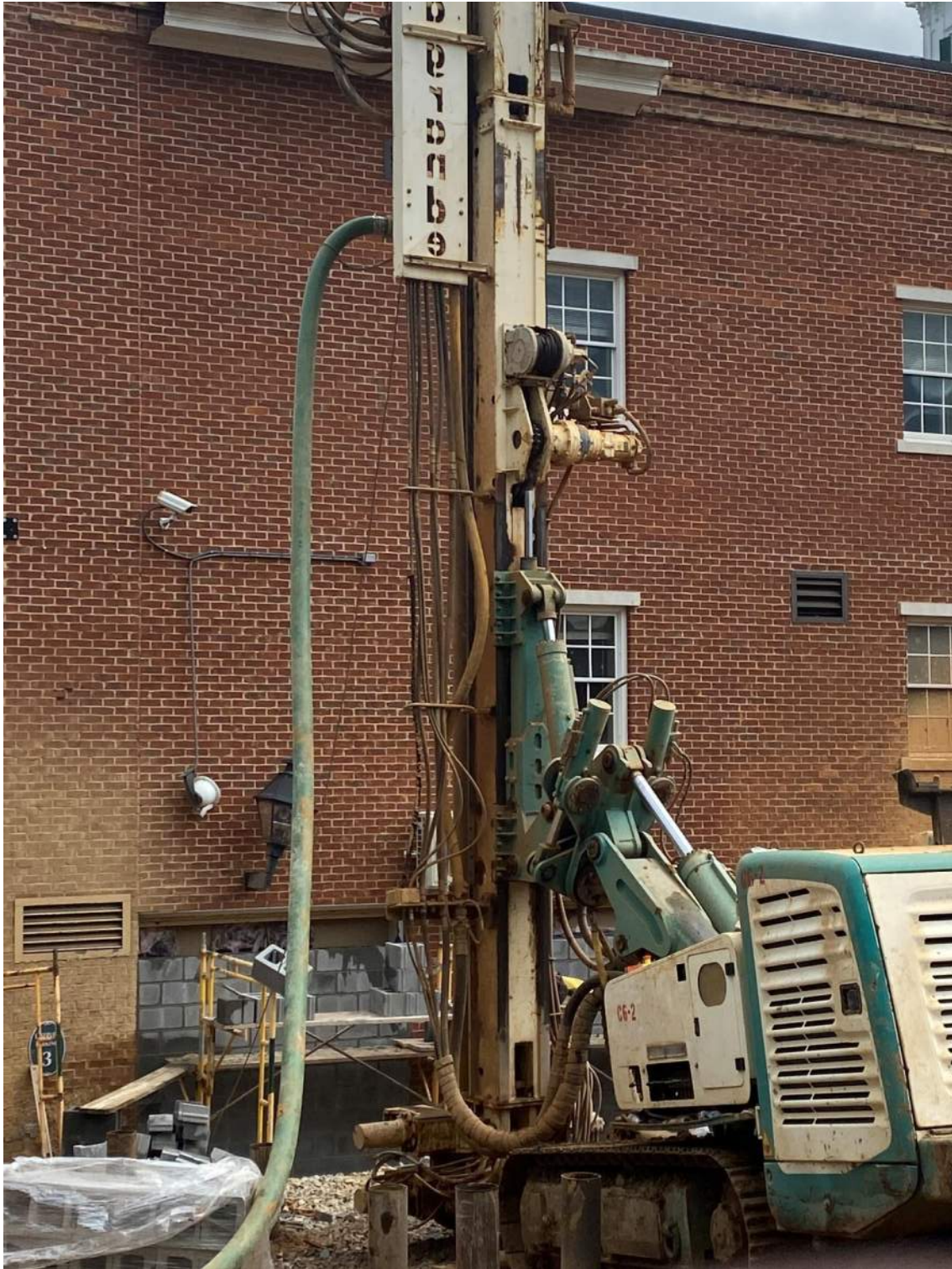
Micro pile installation
