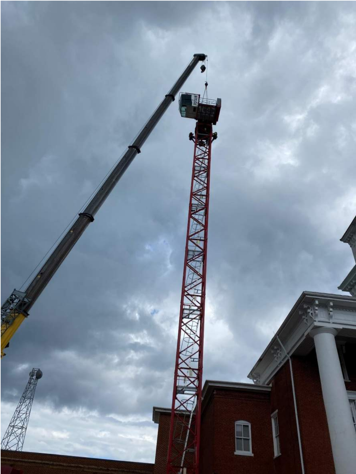
Tower crane installed
