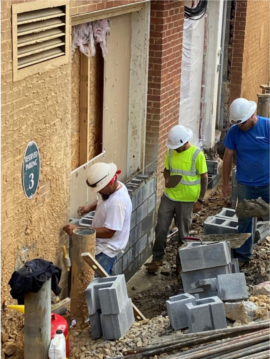
CMU install at old sally port
