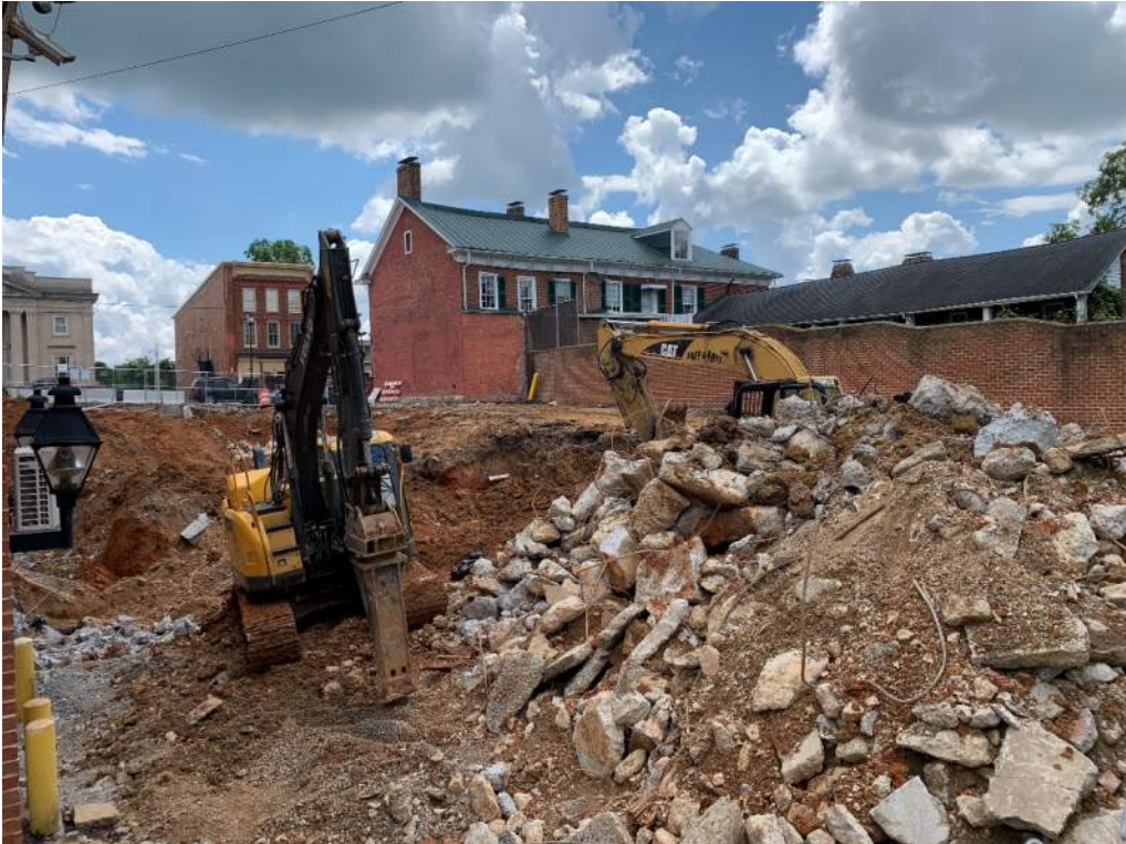
Demolition of old sally port ongoing
