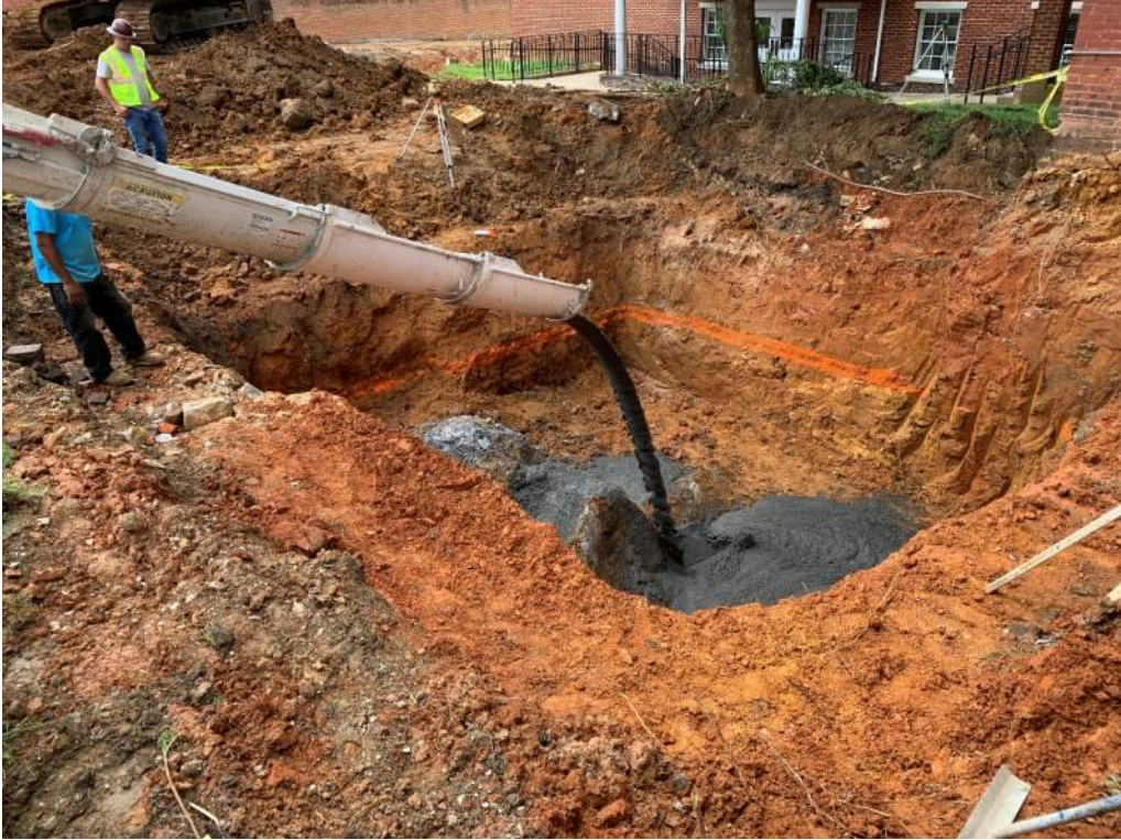
Pouring flow fill at crane foundation undercut
