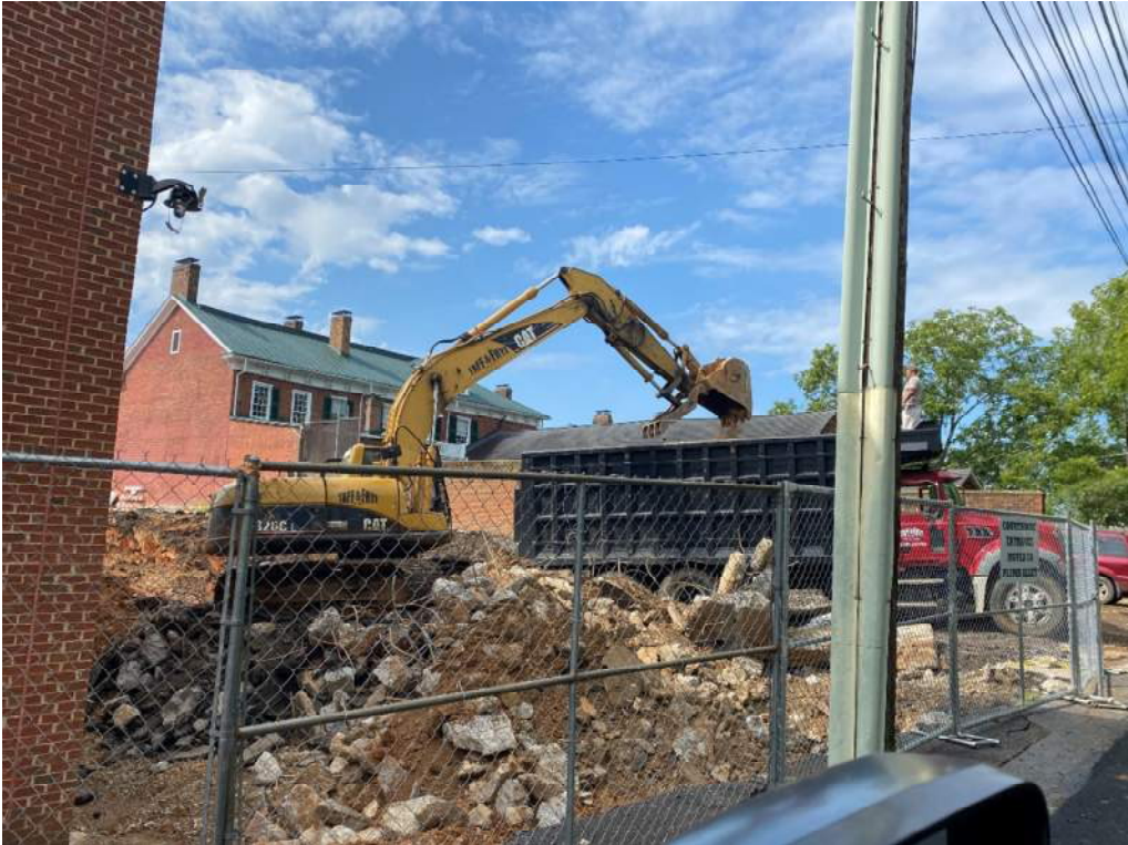
Removal of debris along Plumb Alley
