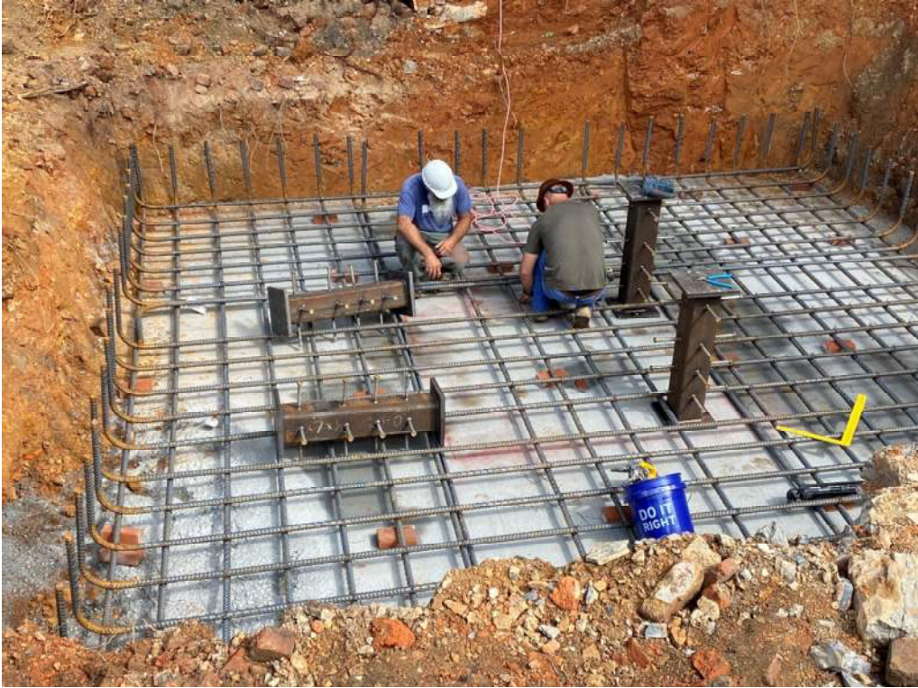
Beam support installation for crane pad foundation
