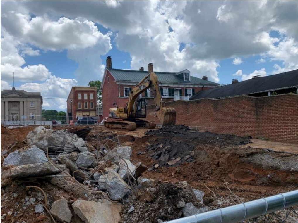
Demolition of asphalt drive off Plumb Alley
