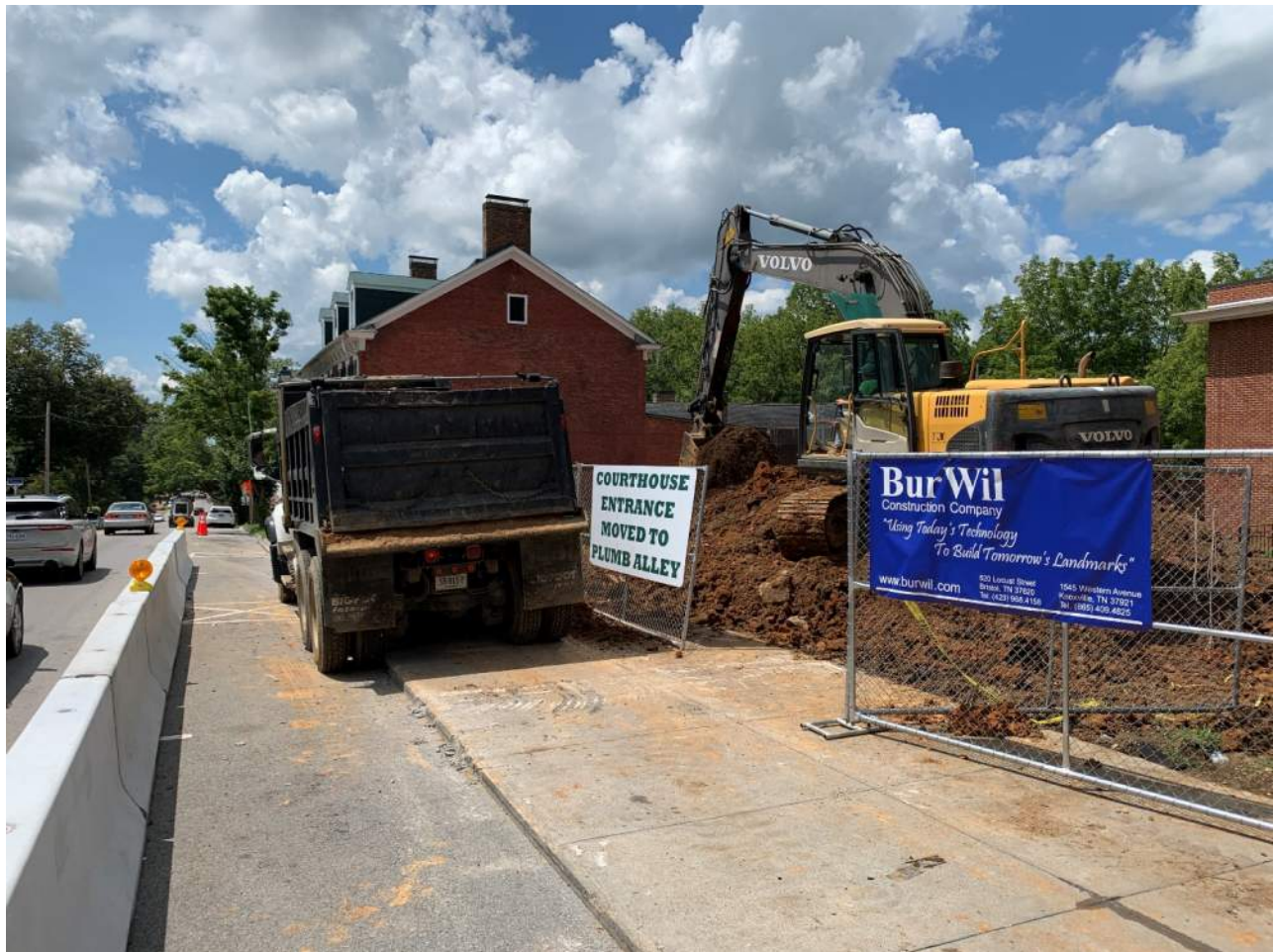
Removal of debris along Main Street
