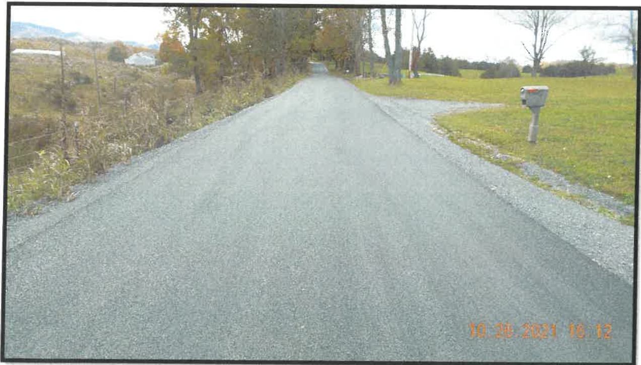
Route 783 – Fairhaven Rd Rural Rustic Project UPC 111419
