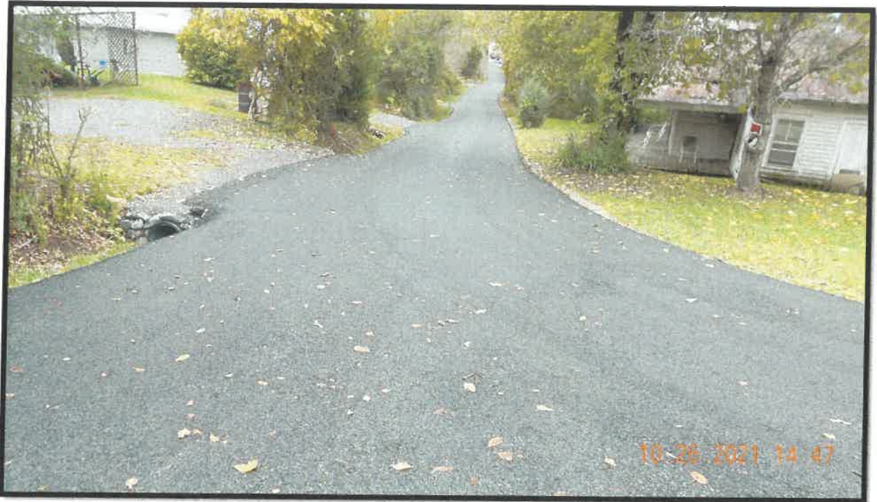
Route 796 – Benfield Lane Rural Rustic Project UPC 111420
