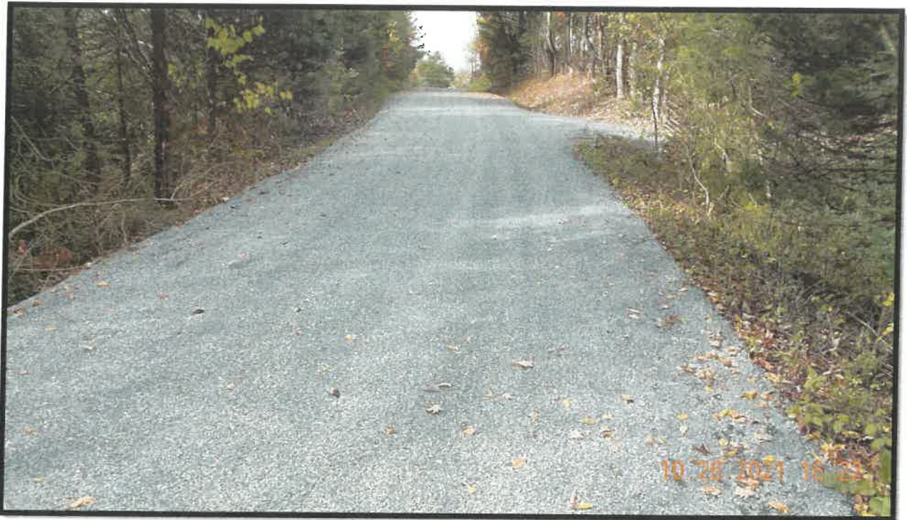
Route 907 – Piper Rd Rural Rustic Project UPC 111770
