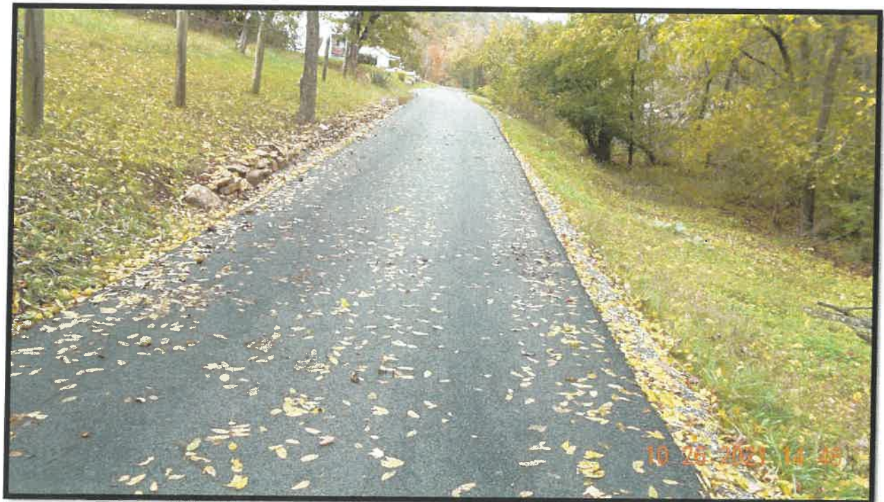
Route 796 – Benfield Lane Rural Rustic Project UPC 111420
