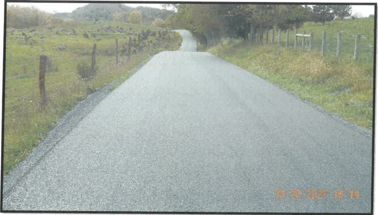
Route 783 – Fairhaven Rd Rural Rustic Project UPC 111419
