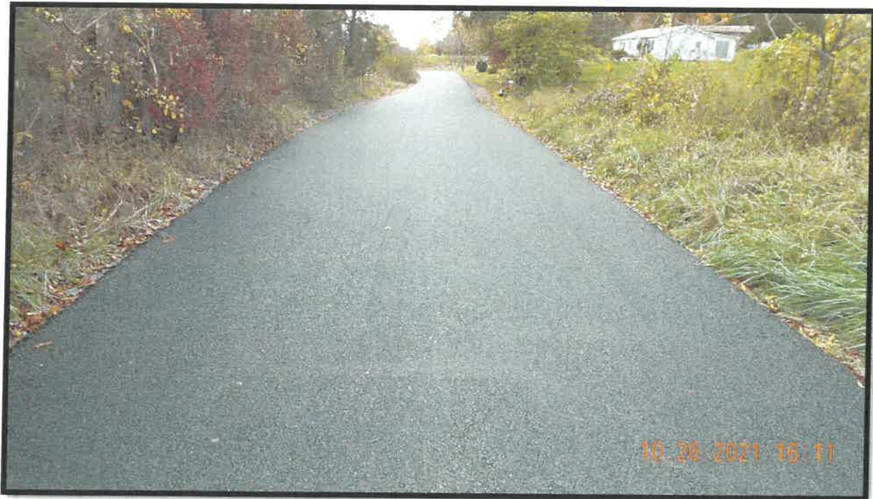
Route 783 – Fairhaven Rd Rural Rustic Project UPC 111419
