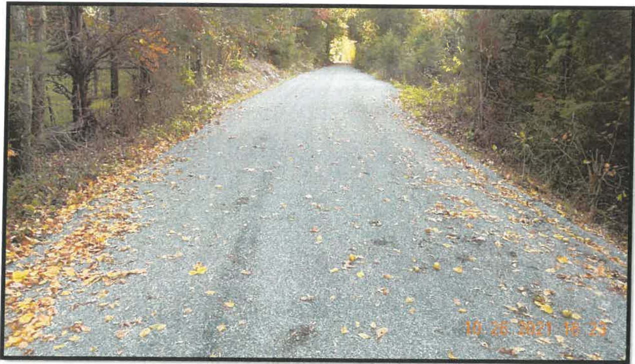
Route 907 – Piper Rd Rural Rustic Project UPC 111770
