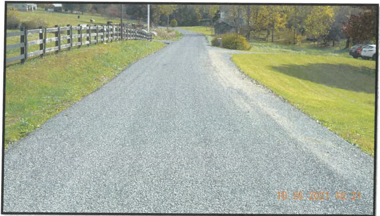
Route 907 – Piper Rd Rural Rustic Project UPC 111770
