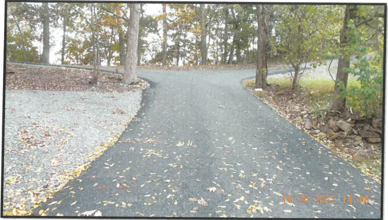
Route 796 – Benfield Lane Rural Rustic Project UPC 111420
