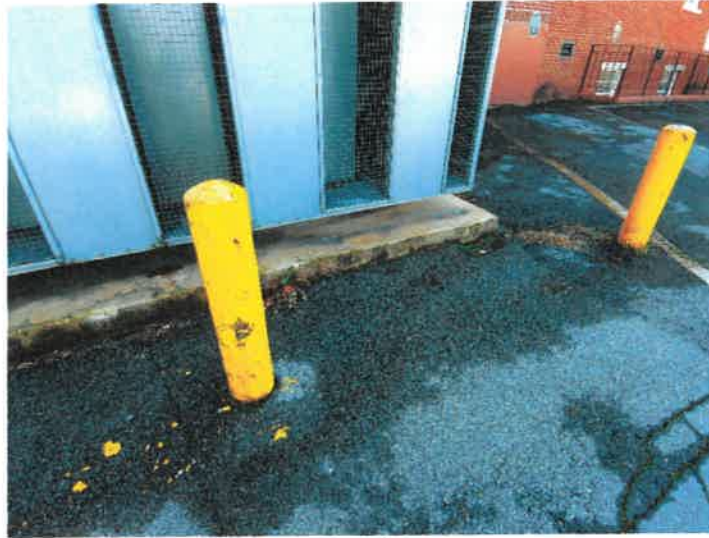
The traffic bollards were found to utilize lead-based paint.
