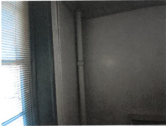
The interior roof drain pipes were found to utilize lead-based paint.
