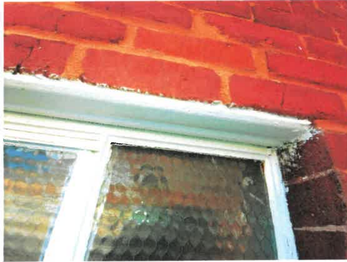
Metal framed basement window components, including lintels, were found to utilize lead-based paint.
