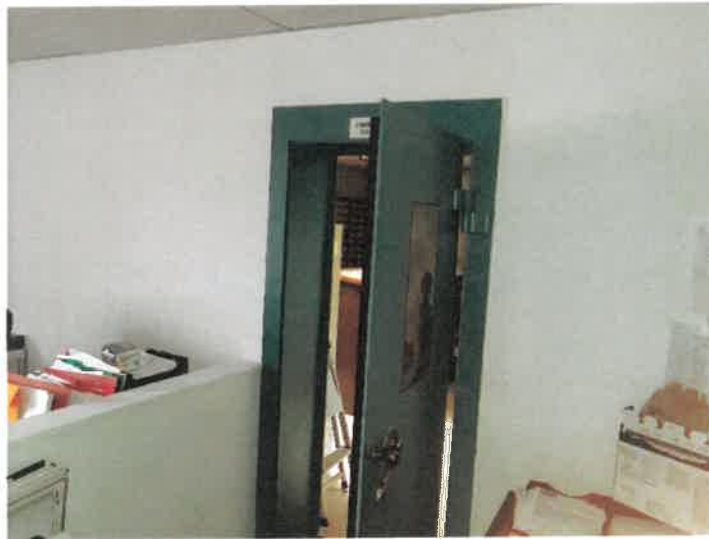
All vault style doors and door casings were found to utilize lead-based paint.
