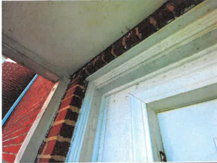
Window and door lintels on the back side of the Elliot Building were found to utilize lead-based paint.
