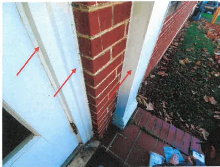
Painted columns and door components on Court Street entrance were found to utilize lead-based paint.
