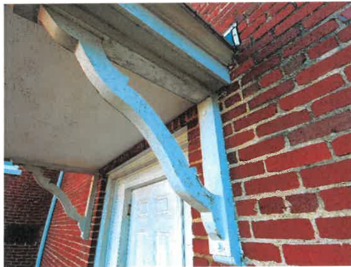
Painted fascia, soffit and trim on the back side of the Elliot Building were found to utilize lead-based paint.
